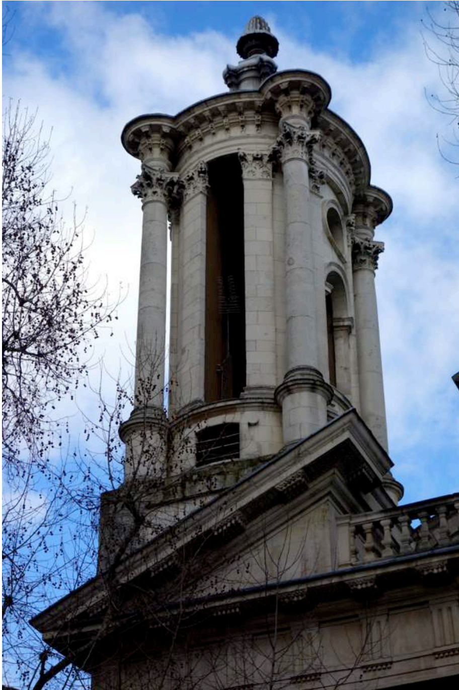
Figure 31. Archer Saint John's Church, Westminster, tower detail 1714-28 Photograph, taken by the author (2015)
