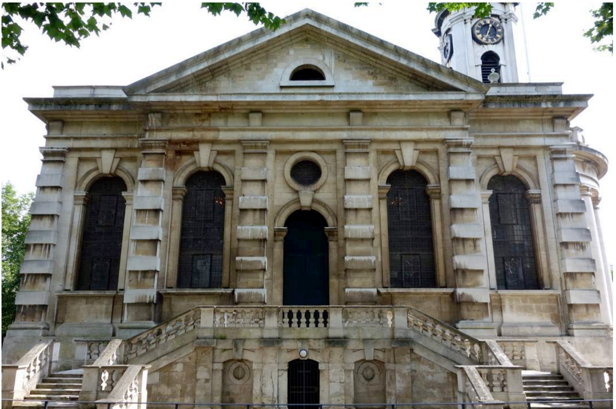
Figure 23. Archer Saint Paul's Church, Deptford, north elevation 1712-30 Photograph, taken by the author (2014)
