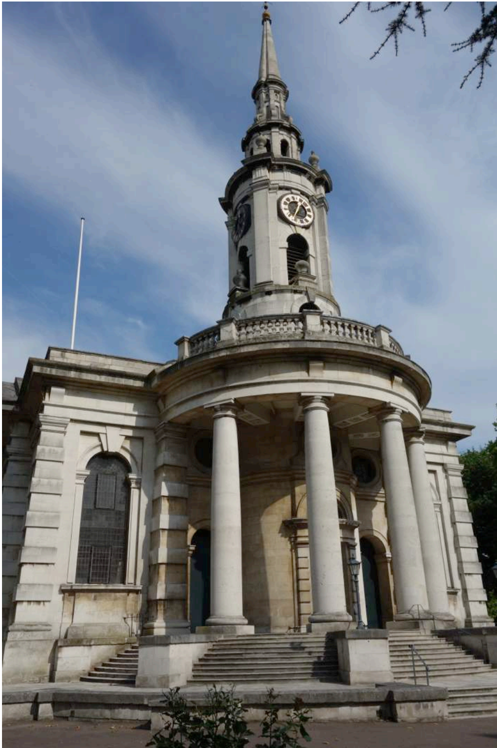
Figure 22. Archer Saint Paul's Church, Deptford, west elevation, tower detail 1712-30 Photograph, taken by the author (2014)
