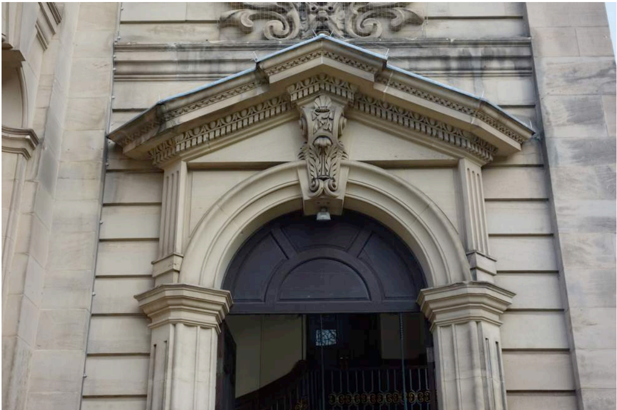
Figure 9. Archer Saint Philip's Cathedral, Birmingham, west entrance, exterior detail 1709-1715 Photograph, taken by the author (2014)
